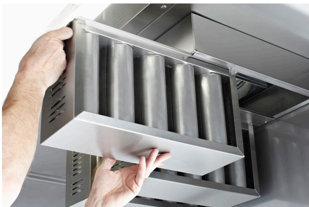
Filterkassetten skyves inn i filterhuset.
